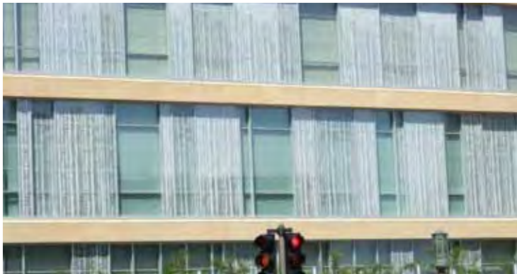
Interior shades and exterior film at the Minneapolis Central Library
