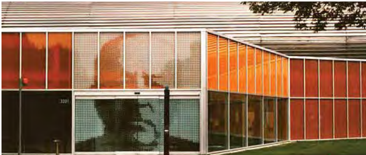
A polycarbonate core makes this glass visible to birds (IIT Student Center, IL)
